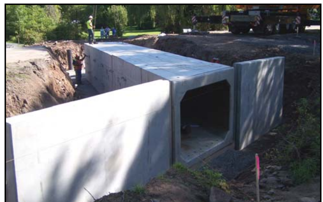
The new box culvert installed on Gordon Road.
