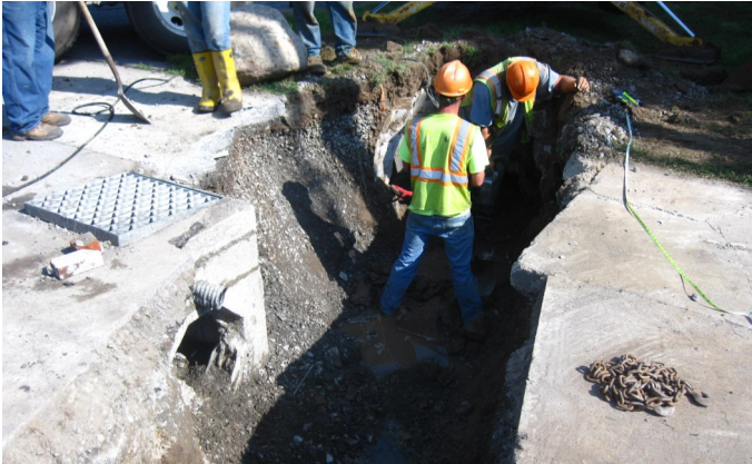
The Sweden highway crew replaces drainage pipe under Sweden Lane in August.
