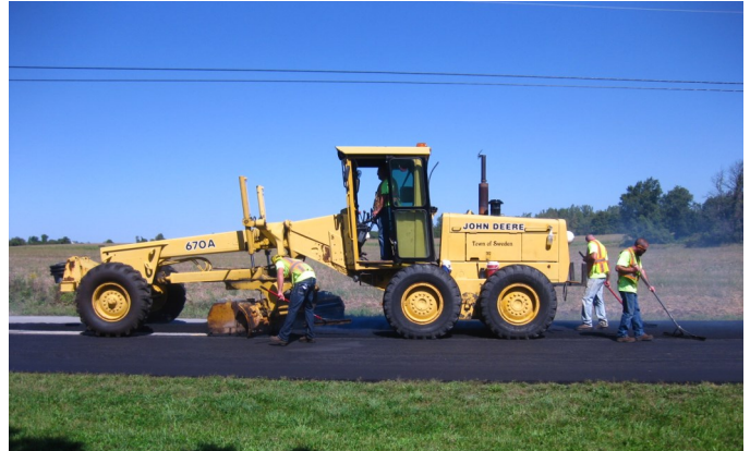
Whittier Road was “trued and levelled” in September in preparation for a repaving project in 2016 or 2017. About 220 tons of asphalt was spread with the town's motor grader.
